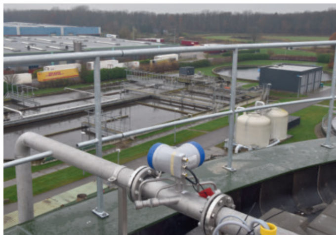
Flow measurement of biogas behind the digester
