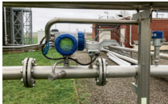
OPTISONIC 7300 Biogas ultrasonic flowmeter and OPTIBAR PM 5060 pressure transmitter installed at the outlet of the digestion tower
