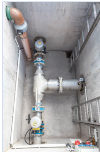
Gauge pressure measurement in an aerator line with the OPTIBAR PM 5060
