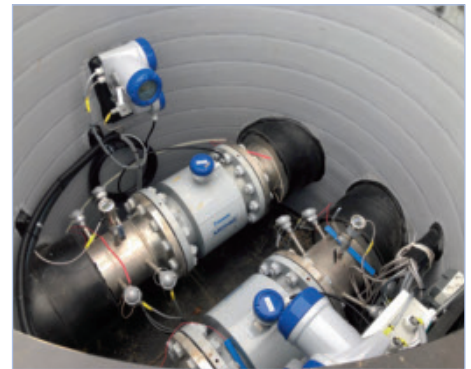
District heating measurement with OPTISONIC 3400 District Heating flowmeter, OPTITEMP TRA-T30 temperature sensor and OPTIBAR PM 3050 pressure transmitter
