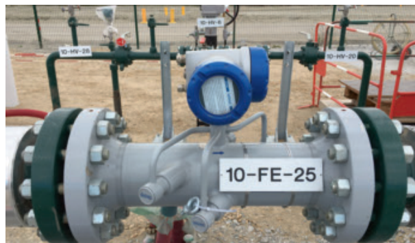
OPTISONIC 7300 ultrasonic flowmeter prior to commissioning
