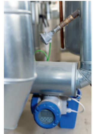
EMF with paired temperature sensor
