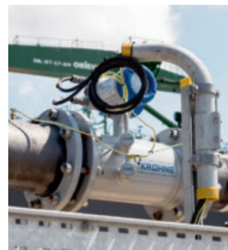
Full bore design of the OPTISONIC 7300 ultrasonic flowmeter
