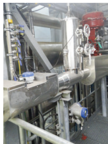
Feedwater measurement with the OPTISONIC 3400 ultrasonic flowmeter
