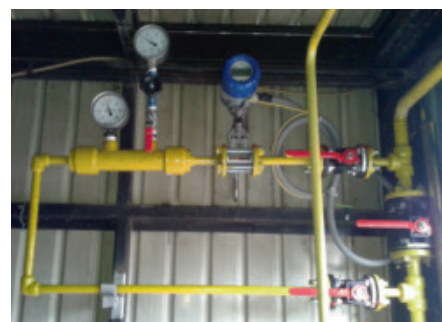
Vortex flowmeter mounted in a bypass line
