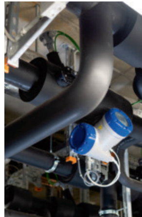
Electromagnetic flow measurement of hot water
