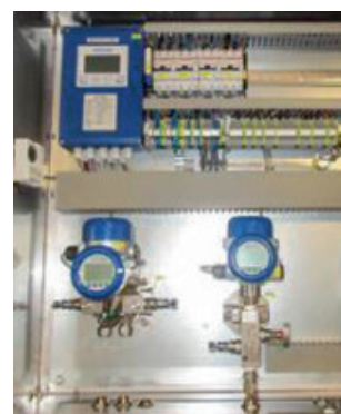
Control cabinet with KROHNE DP and pressure transmitters, temperature transmitter and flow computer
