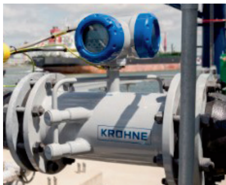
Ultrasonic flow measurement of hydrocarbon vapors
