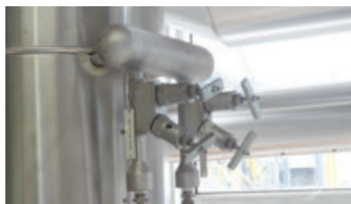
Venturi nozzle installation
