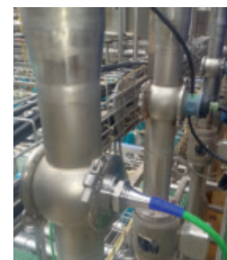
Inductive conductivity measurement of cleaning agents
