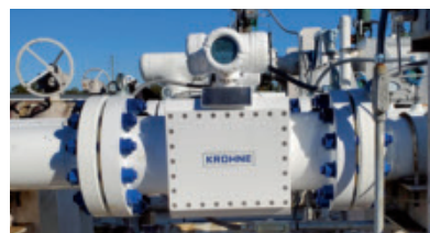
Custody transfer flow measurement of natural gas
