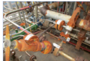
Retrofitted flange pressure tapping
