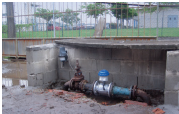
Use of WATERFLUX in partially flooded areas
