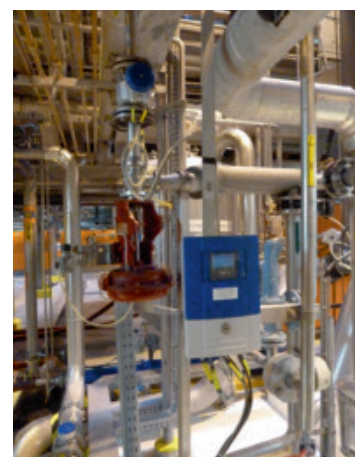
Electromagnetic flowmeters on water circuits
