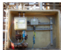
Previous DP transmitter before replacement
