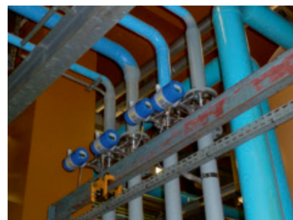
Vortex flowmeters measuring compressed air
