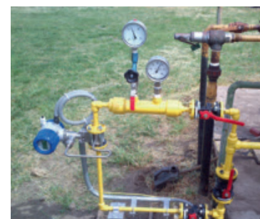
Installation of flowmeter with sandwich connection
