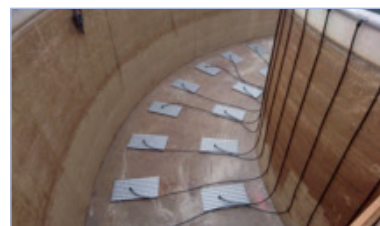
Aeration elements of an aeration basin
