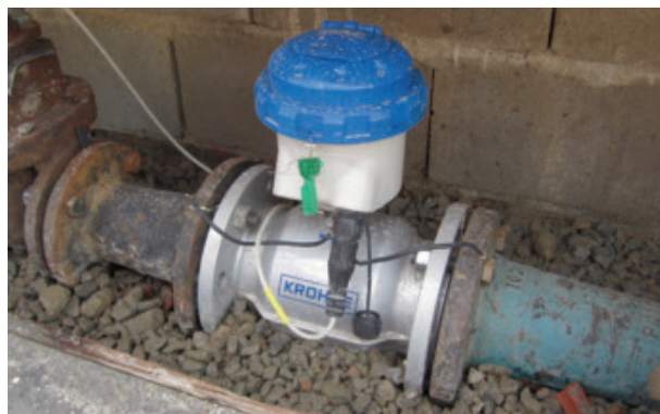
Measuring tube supported by gravel bed
