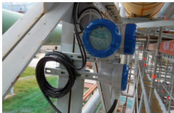
OPTISONIC 8300 ultrasonic flowmeter
